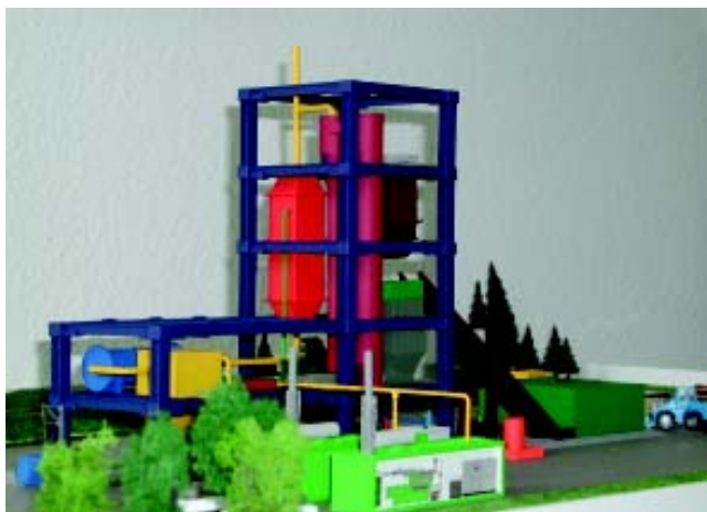
Pre-commercial demonstration plant with 5.0 MW fuel input, corresponding to 1.45 \text{ MW}_{\text{el}}
