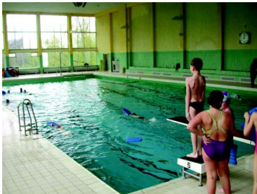
Electrolysis for water disinfection at the public pool at Lünen
