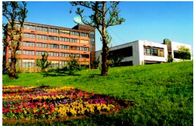
The Fraunhofer Institute for Environmental, Safety, and Energy Technology UMSICHT
