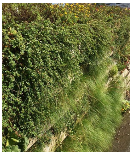
Pilotwand in Castrop-Rauxel.
