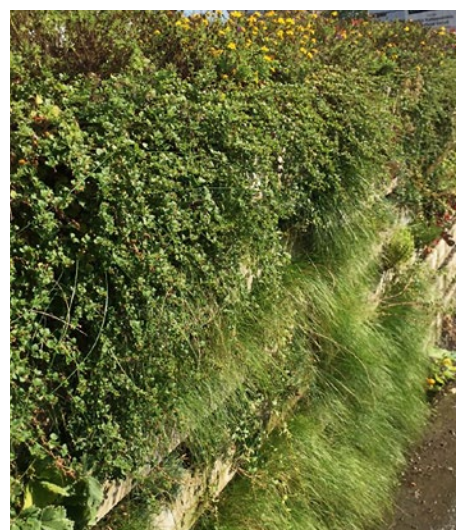
Pilot wall in Castrop-Rauxel.
